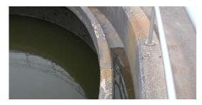
The concrete wastewater tanks were first sandblasted and then pressure washed to remove all loose material. Exposed rebar was coated with patent pending MCI® 2023. This passivating repair grout gives extra corrosion protection to reinforcing steel for long term resistance. Spalled areas were repaired with MCI® 2038, a two component, fiber-reinforced finish repair mortar. The entire surface of the tanks were treated with MCI® 2020, NSF Standard 61 approved for potable water applications.
